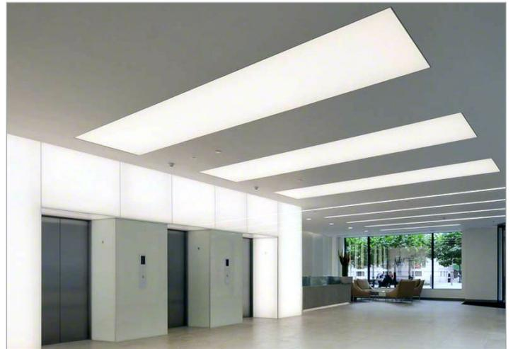
Lighting for ceiling panels can be controlled with 'intelligent' auto-dimming features, colour-change capabilities and more. Using different colour-temperature white LEDs, it's possible for bright, cool illumination during the day to gradually change to warmer, softer light as the evening progresses.
